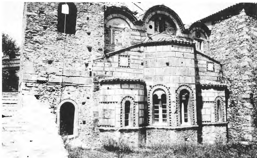
Fig. 2. Mistra. Metropolis (St. Demetrius), east facade. The level of the original roof is clearly indicated by the arch immediately above the main apse and the corresponding, oblique lines of roof tiles above the lateral apses (photo: H. Torp).
